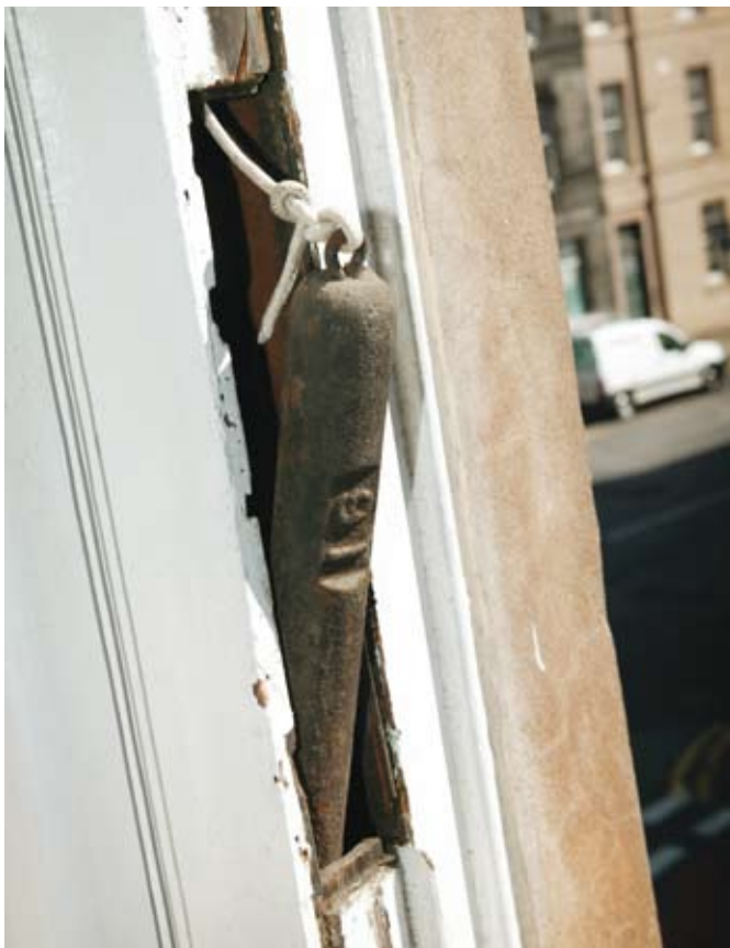
The sash weight can be seen here where the pocket piece has been removed to expose the interior of the window case.
