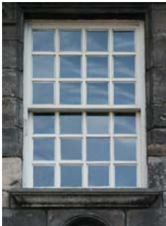
An early sash and case window with thick astragals
