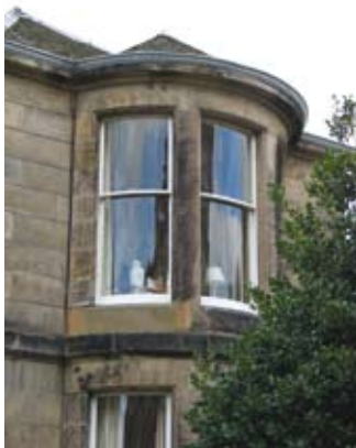
A fine example of 19th Century curved sash frames and glass
