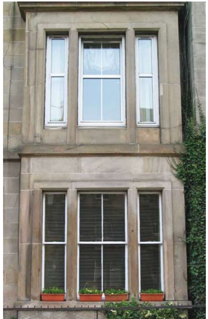
Replacing traditional sash and case windows changes the character and appearance of a building.
